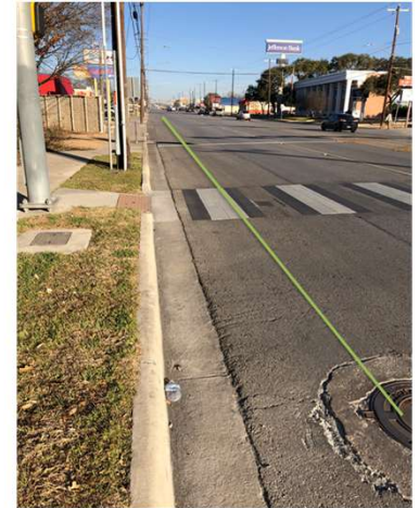
• Looking North along Sewer Main at Fred. Rd
